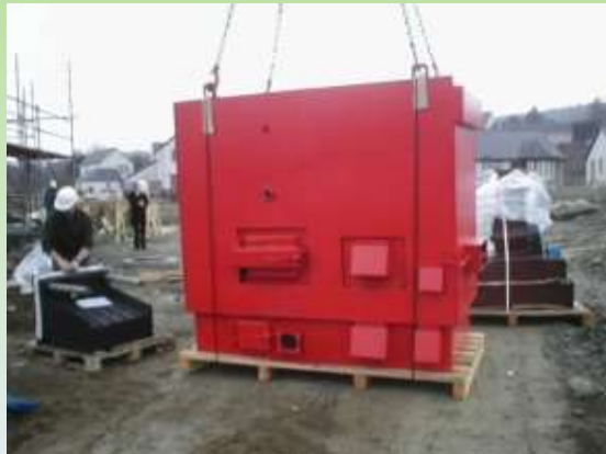
Lynn Road biomass boiler being delivered
