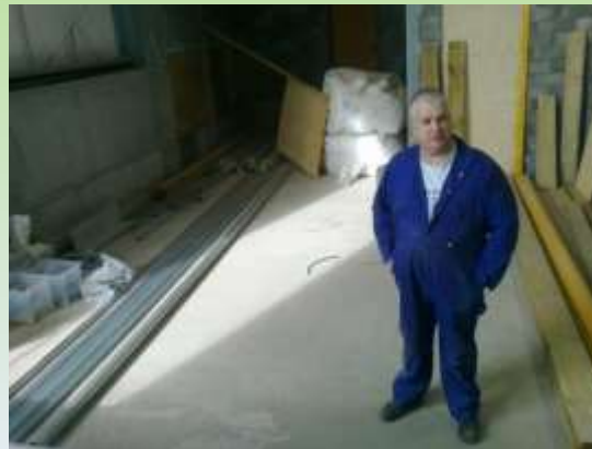
80 m 2 floor under construction
